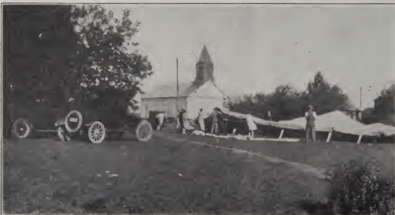
ERECTING THE TENT AT THE MISSION HOUSE CONFERENCE AFTER THE STORM LAST YEAR
